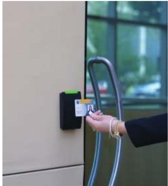
The Access Control System itself also offers redundancy in that the access controllers along with the controlled doors, continue to operate without any local degradation in operation or security, even if there is a power failure (for at least 8 hours) or network failure. Culminated with comprehensive training, operators of the system found it to be user friendly, simple to grasp and most certainly comprehensive with many features.
